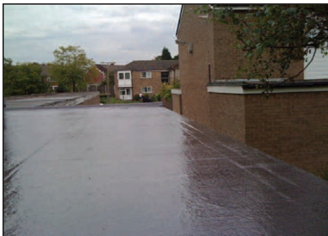
After AFM Roof
