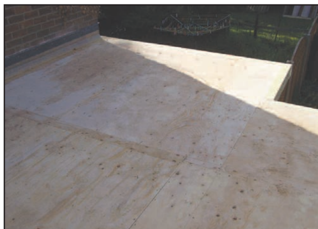
New plywood deck fitted
