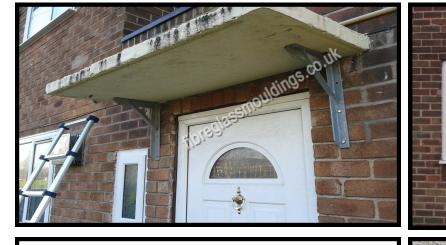
The steel brackets have been designed for additional support and concealed with GRP decorative legs. They are also designed to withstand both snow loading / maintenance
